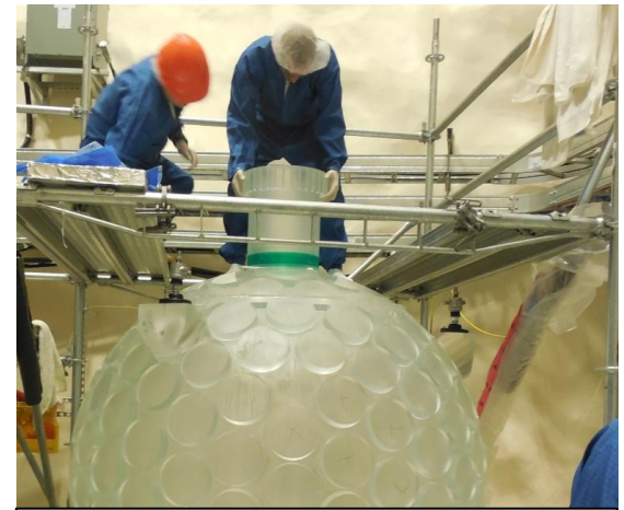
Neck bonding at SNOLAB
