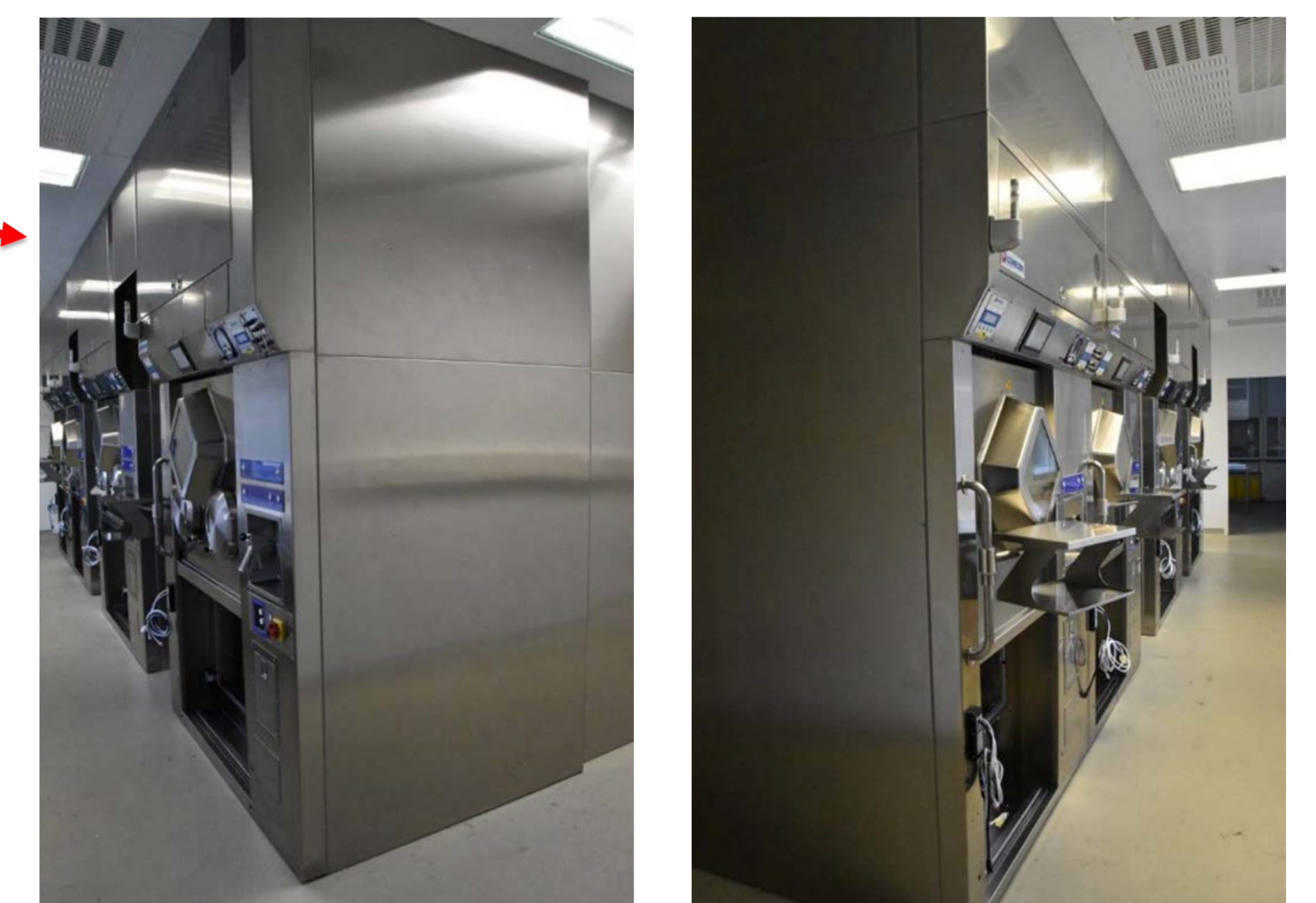
Hot cells in the GPM-lab
