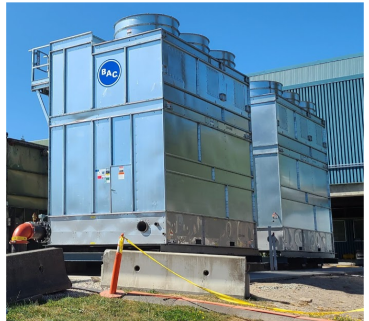
Cooling Tower replacement
