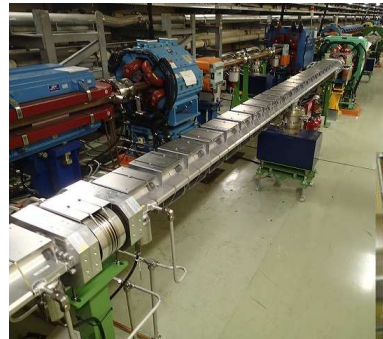
Magnet units attached to beam pipes
