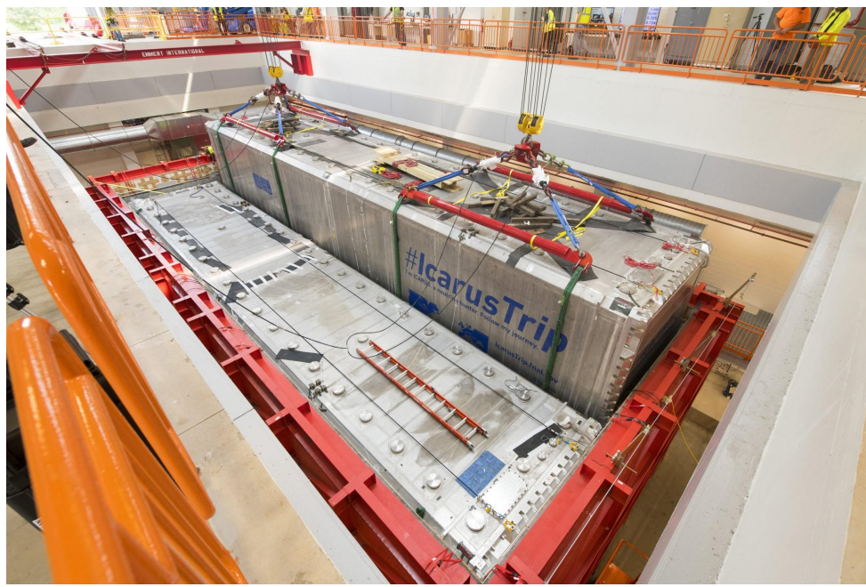
Installing second cold vessel (August 14, 2018)
