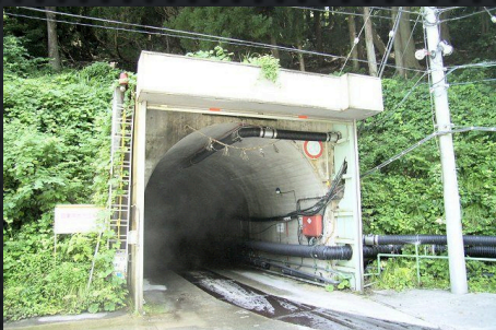
Entrance of the 2km horizontal tunnel
