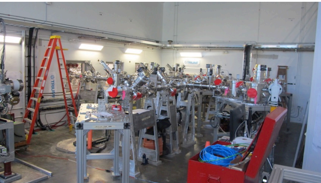
ARIEL Building, ground floor
