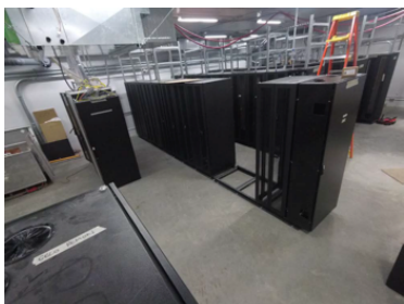
B1-Level Racks installed
