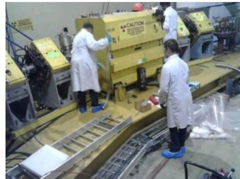
BL4N vault installation
