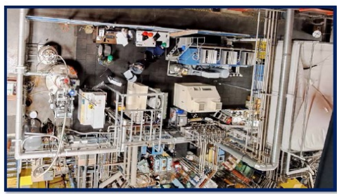
Current view of liquefier cage
