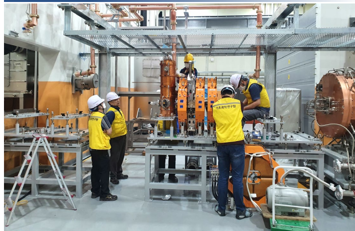
Jul, 2020: Installation of MEBT
