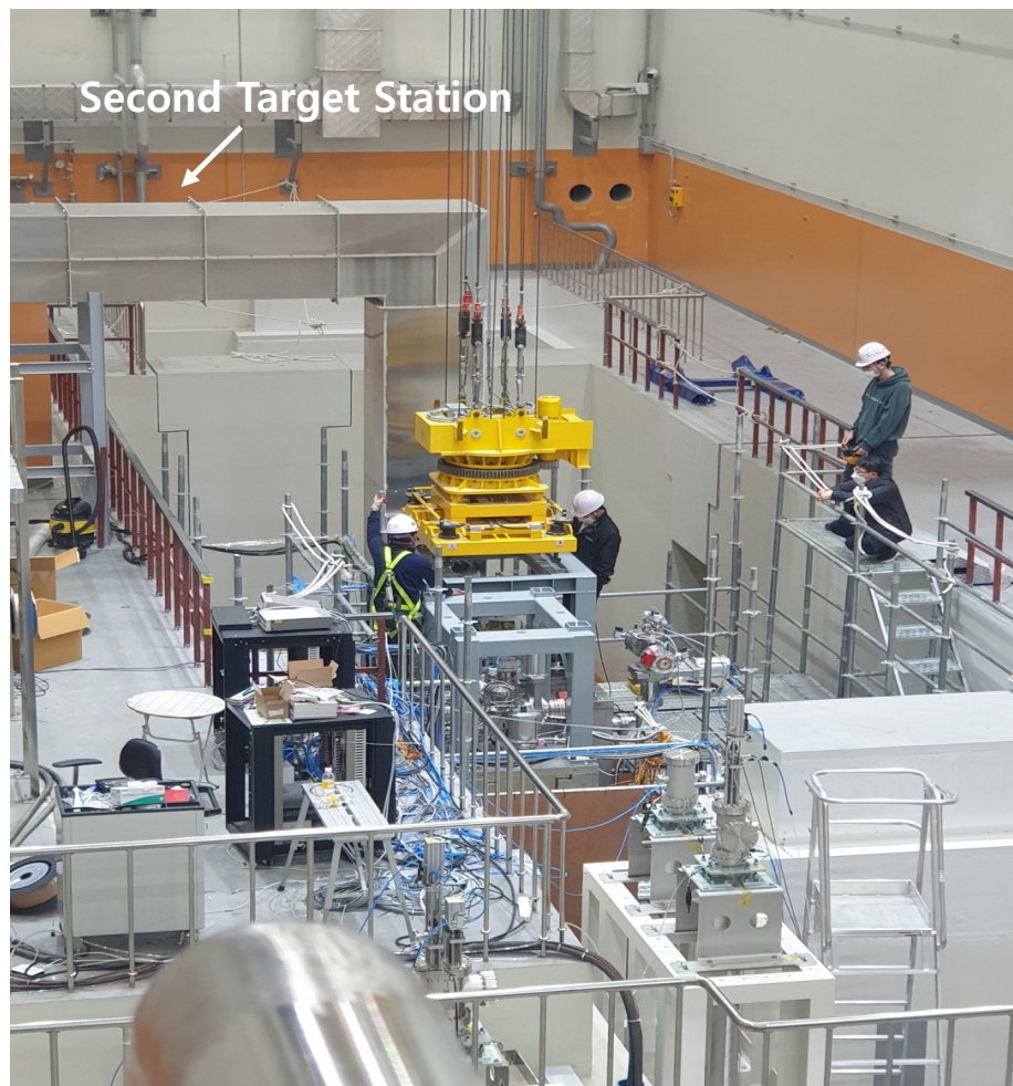
Oct. 2021 Installation of ISOL TIS
