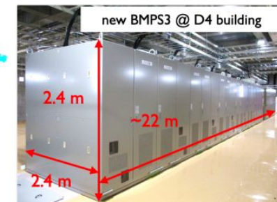
New Power Supply for MR main magnets
