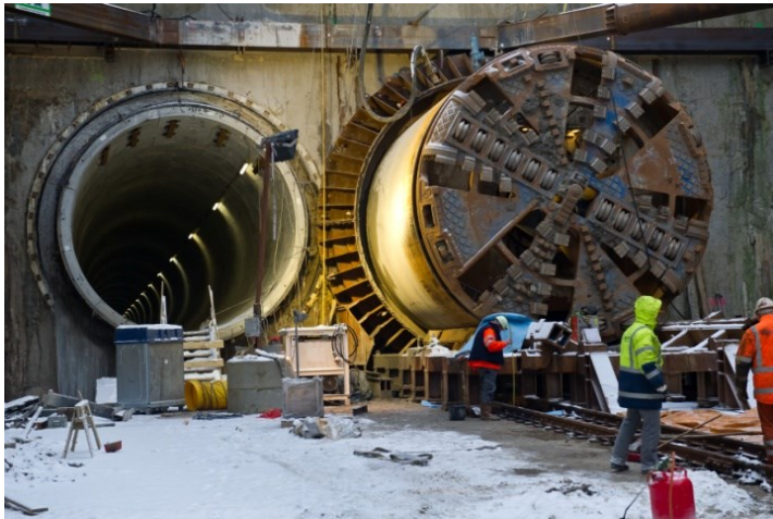
Breakthrough at beam switchyard
