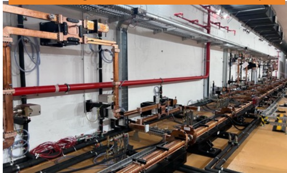
Accelerating structures in Accelerator Bay 2
