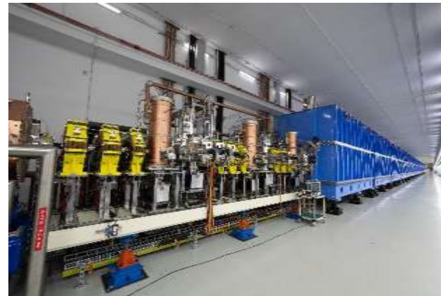
iLinac was installed into tunnel in Sept. 2025
