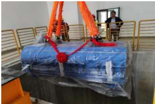
The first dipole was moved into the tunnel in 27 th March, 2024
