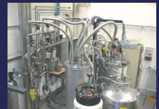
T Calibration station
