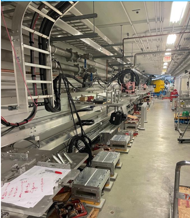
Tunnel beamline, magnets and services
