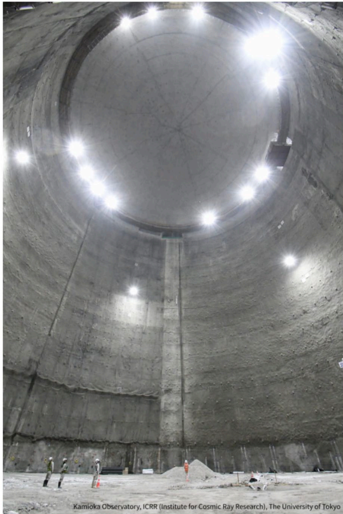
The main Hyper-Kamiokande cavern after excavation completed
